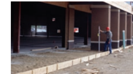
Forms and Footings
