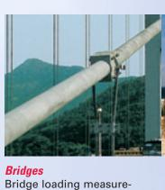
ments, permanent deformation measurement, automatic observation of the bearing pads.
