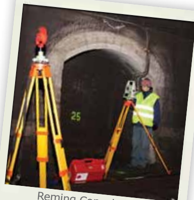
Reming Consult a.s., Zameranie žel. tunela
