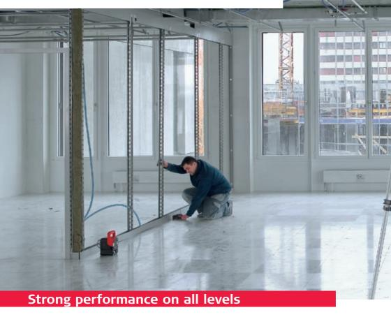
The impressive features of the Leica Roteo 35 include: The integrated motorised wall mount quickly adjusts the laser height to precise accuracy with the remote control. Horizontal and vertical lines or an exact 90° angle – it is no problem for the Leica Roteo 35. The rotating laser can automatically self-level for inclined set-ups of up to  $\pm$  4.5°.
